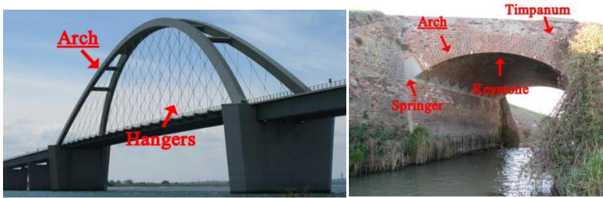
Figure 26. On the left, a through arch bridge: Fehmarnsund Bridge in Germany - Source: [12] On the right, a masonry bridge: Ponte di Aselogna – Source: [14]
