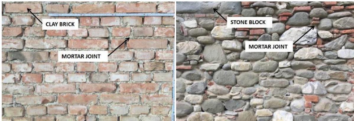
Figure 2. Example of masonry typologies - Source: [2]
