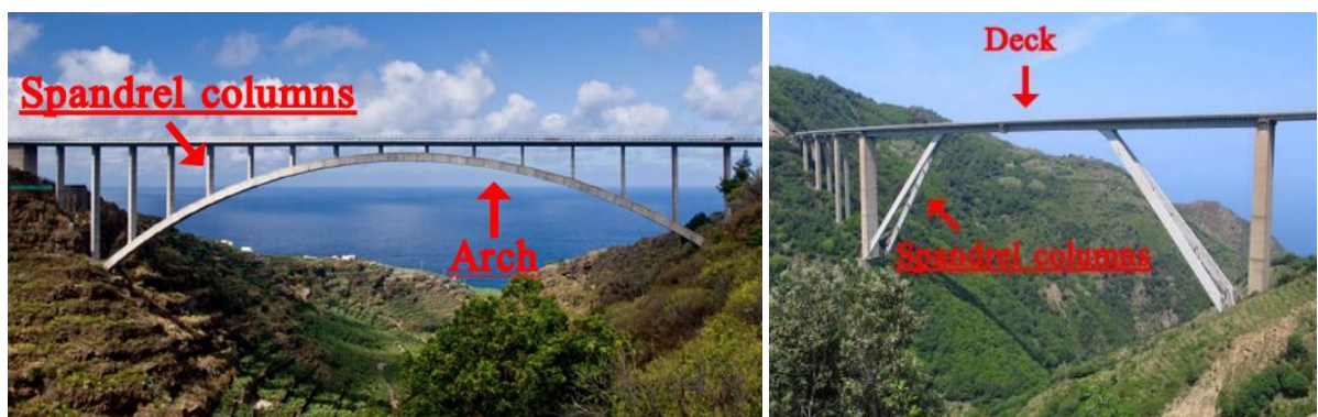
Figure 40. On the left, Los Tilos bridge, La Palma, isole Canarie – Source: [13]. On the right, Viadotto Sfalassà, Bagnara Calabria, Calabria – Source: [11]
