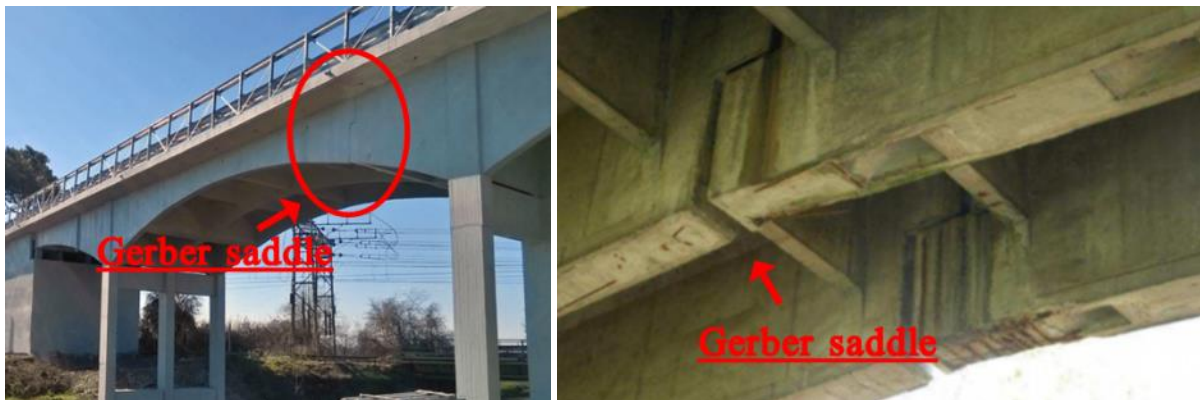
Figure 33. Gerber saddles – Source (left): [26]. Source (right): [27]
