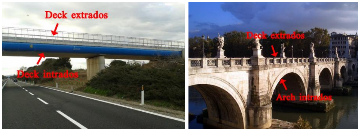
Figure 35. On the left, Cavalcavia s.s. Aurelia – Source: [30]. On the right, Ponte Sant’Angelo, Roma – Source: [31]
