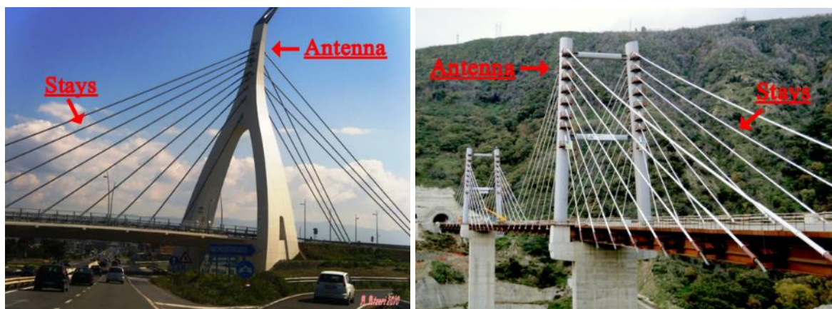
Figure 24. On the left, cable-stayed bridge Emanuela Loi, Monserrato, Sardegn – Source: [10]. On the right, Viadotto Favazzina, Bagnara Calabria-Scilla, Calabria – Source: [11]
