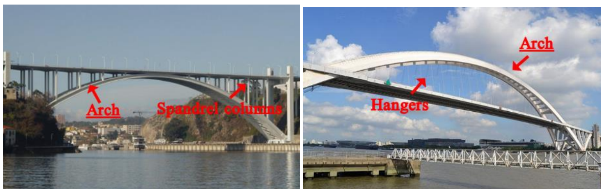
Figure 25. On the left, a deck arch bridge: Ponte Arrabida, Porto - Source: [12]. On the right, a half-trough arch bridge: Lupu Bridge, China. Source: [13]
