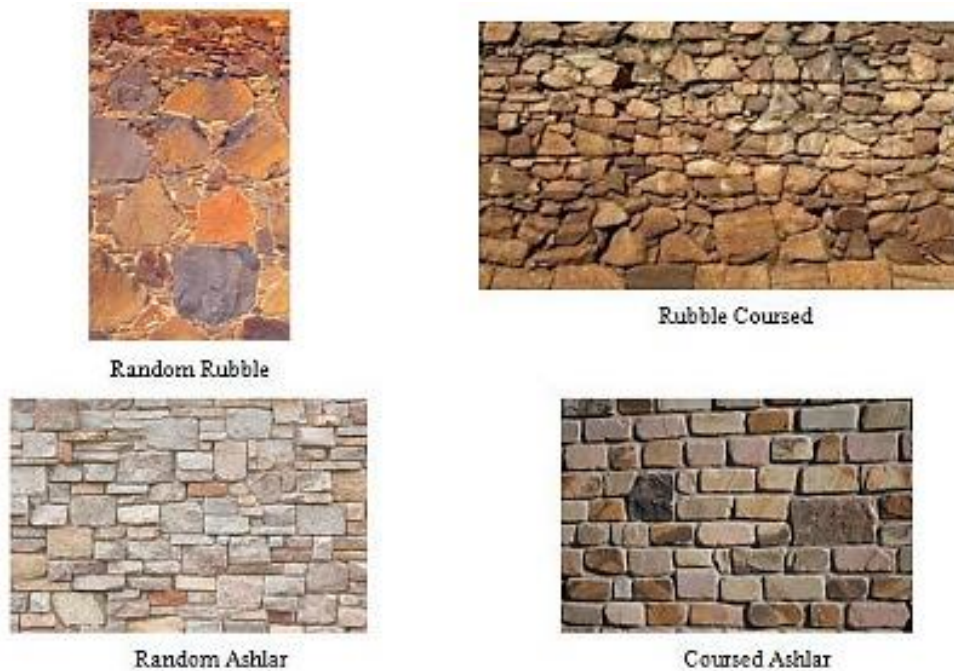
Figure 3. Examples of stone bond - Source: [3]
