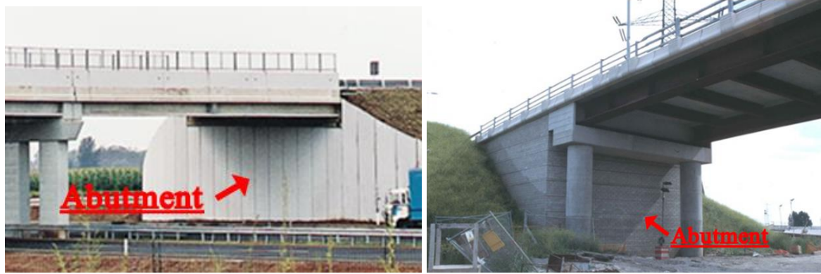
Figure 23. Bridge abutment – Source (left): [8]. Source (right): [9]
