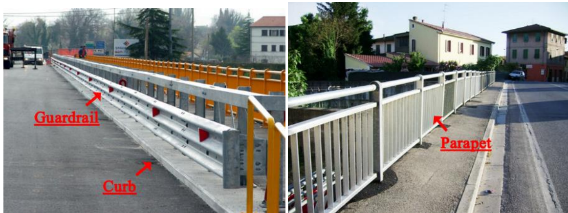
Figure 29. On the left, an example of bridge with curb and guardrail – Source: [18]. On the right, an example of bridge with parapet - Source: [19]
