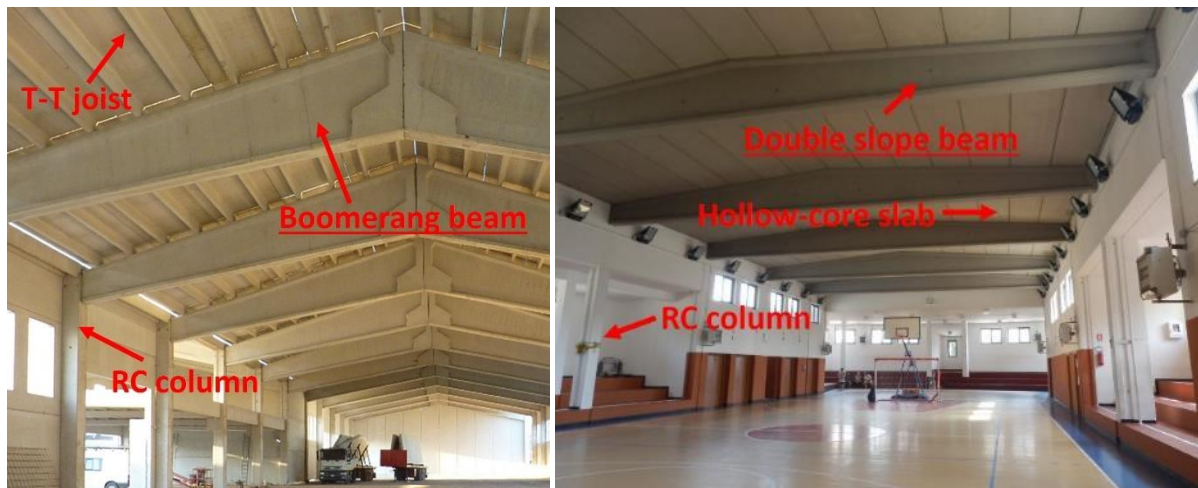
Figure 48. On the left, roof with boomerang beam – Source: [37]. On the right, roof with double slope beam – Source: [7]
