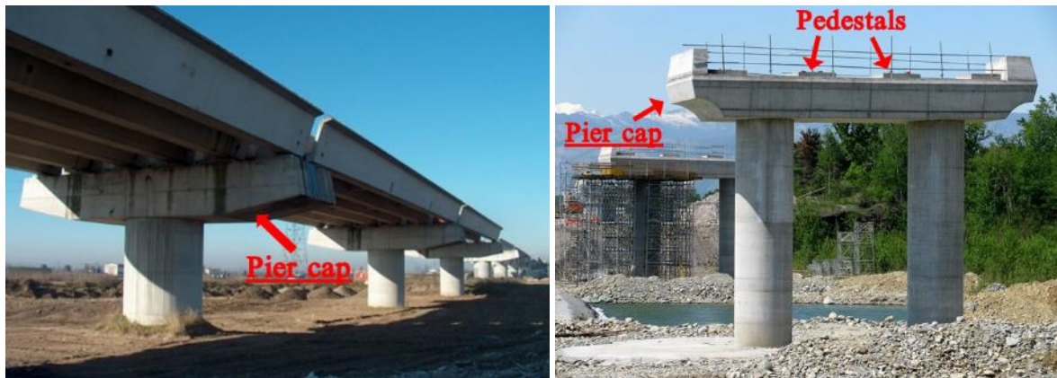
Figure 39. On the left, pier cap on single column – Source: [35]. On the right, multiple columns and pier cap. – Source: [8]
