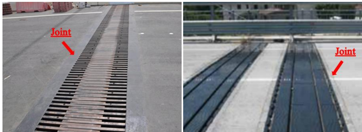
Figure 36. Expansion joint – Source: [32]
