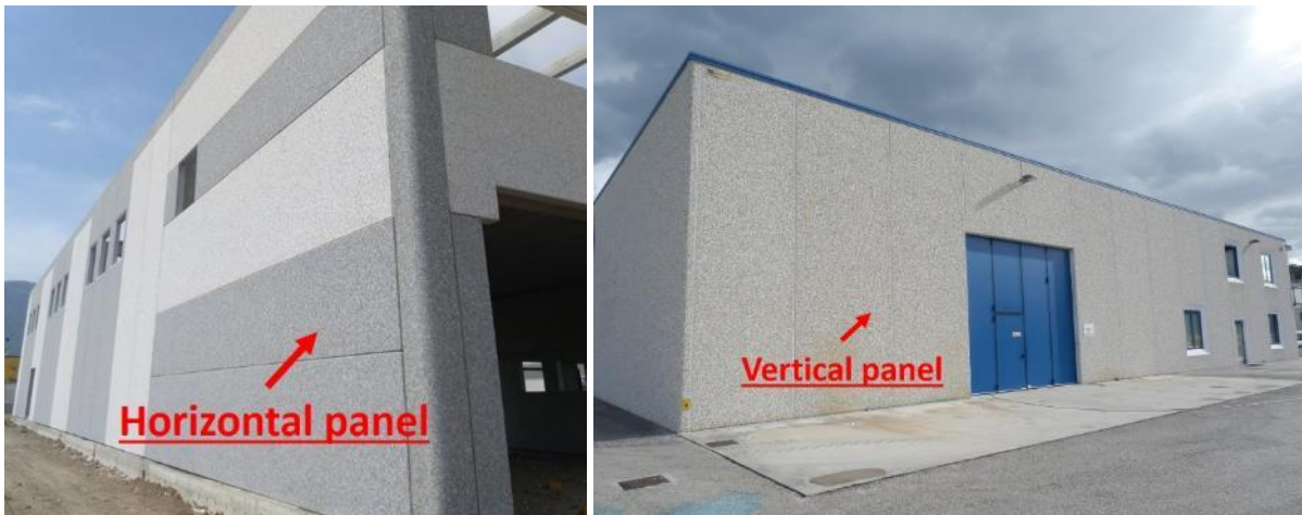
Figure 52. On the left, horizontal panels – Source: [38]. On the right, vertical panels – Source: [7]
