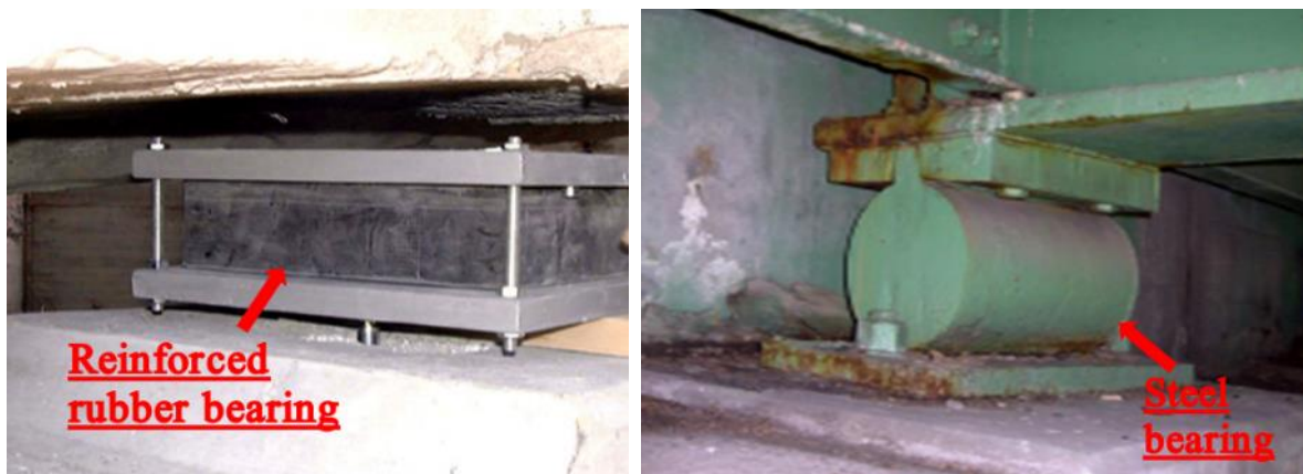
Figure 28. Close view of a rubber bearing with anchor plate (left) and a steel bearing (right) – Source: [17]
